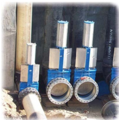
Mixing chamber installation
